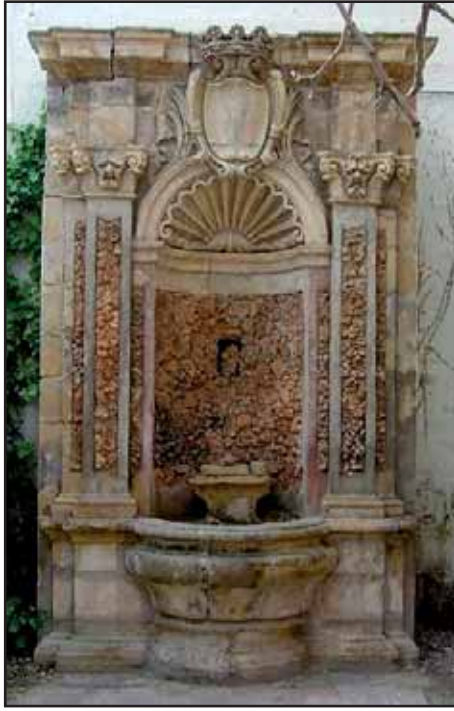
Consolidation and restoration of masonry surface
