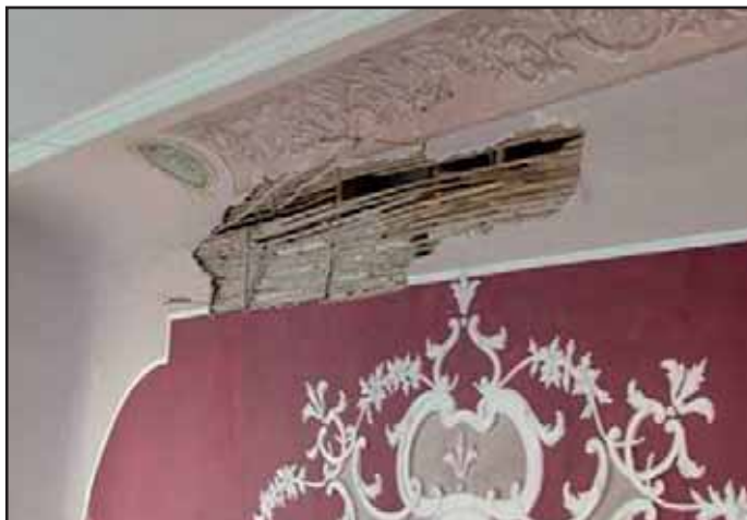
Exposed bamboo soffit
