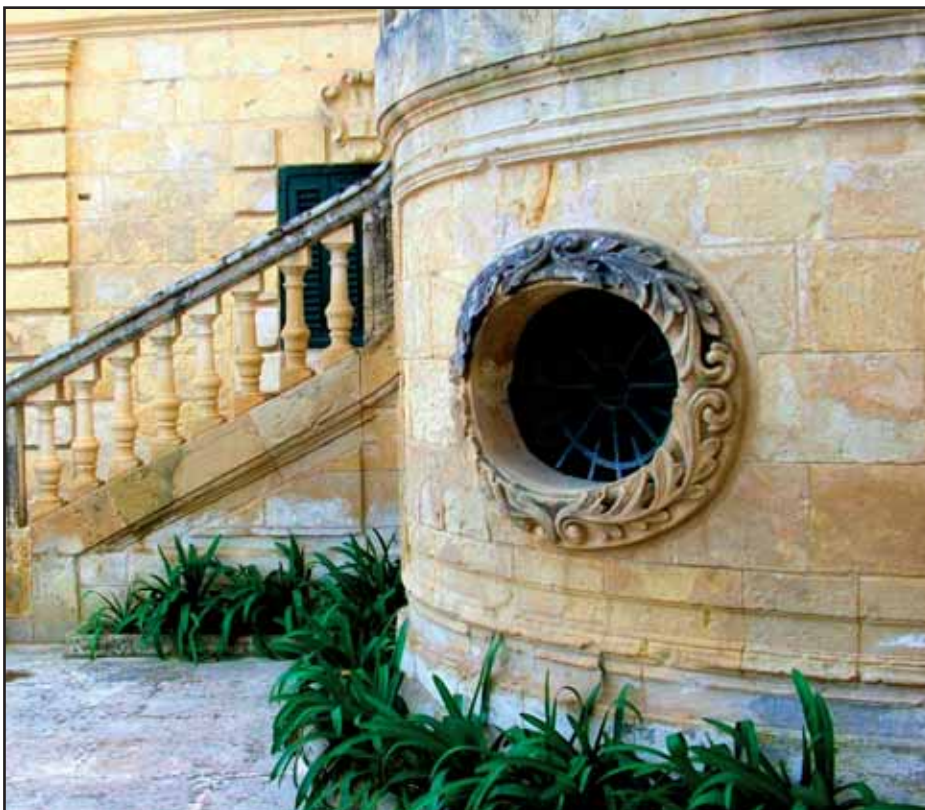
Detail of external staircase
