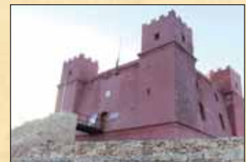
St Agatha's Tower commonly known as the Red Tower, Mellieha, built in 1647/48 by Grand Master Jean Paul Lascaris Castellar - Restored in 2001.
