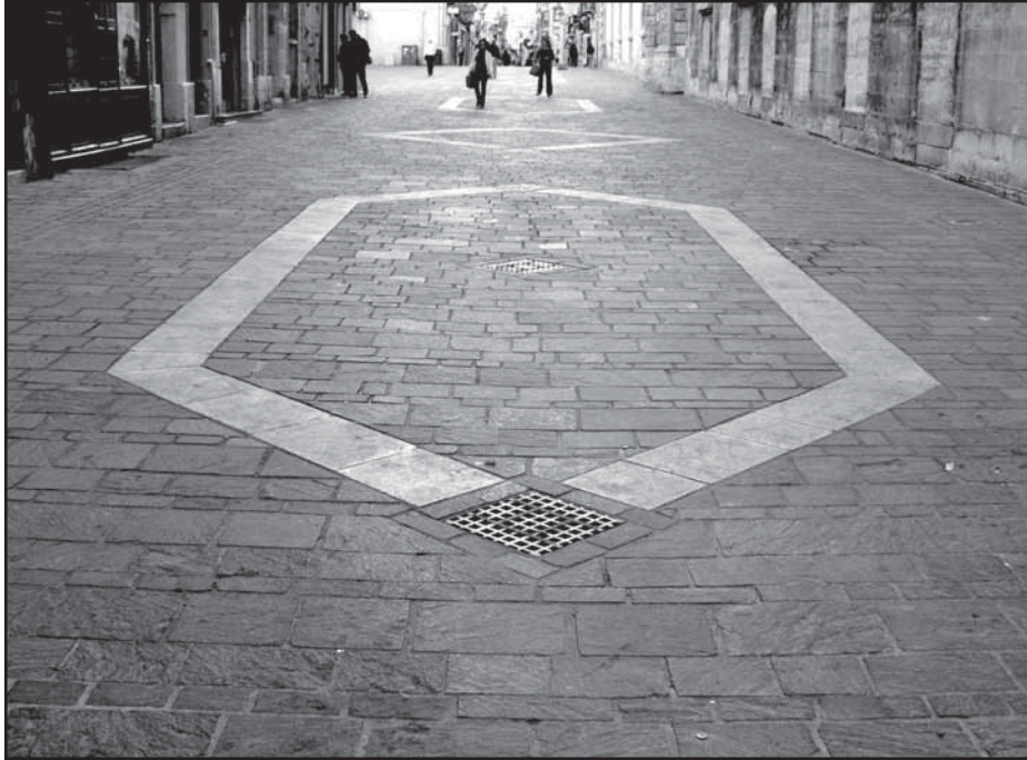
Paving in Merchants Street
