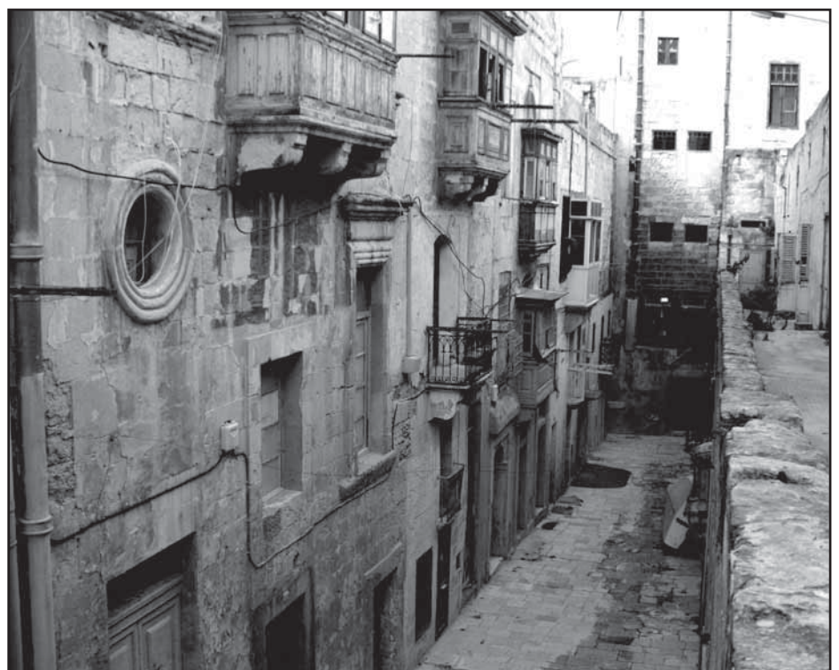
Derelict buildings in the Bicċerija area
