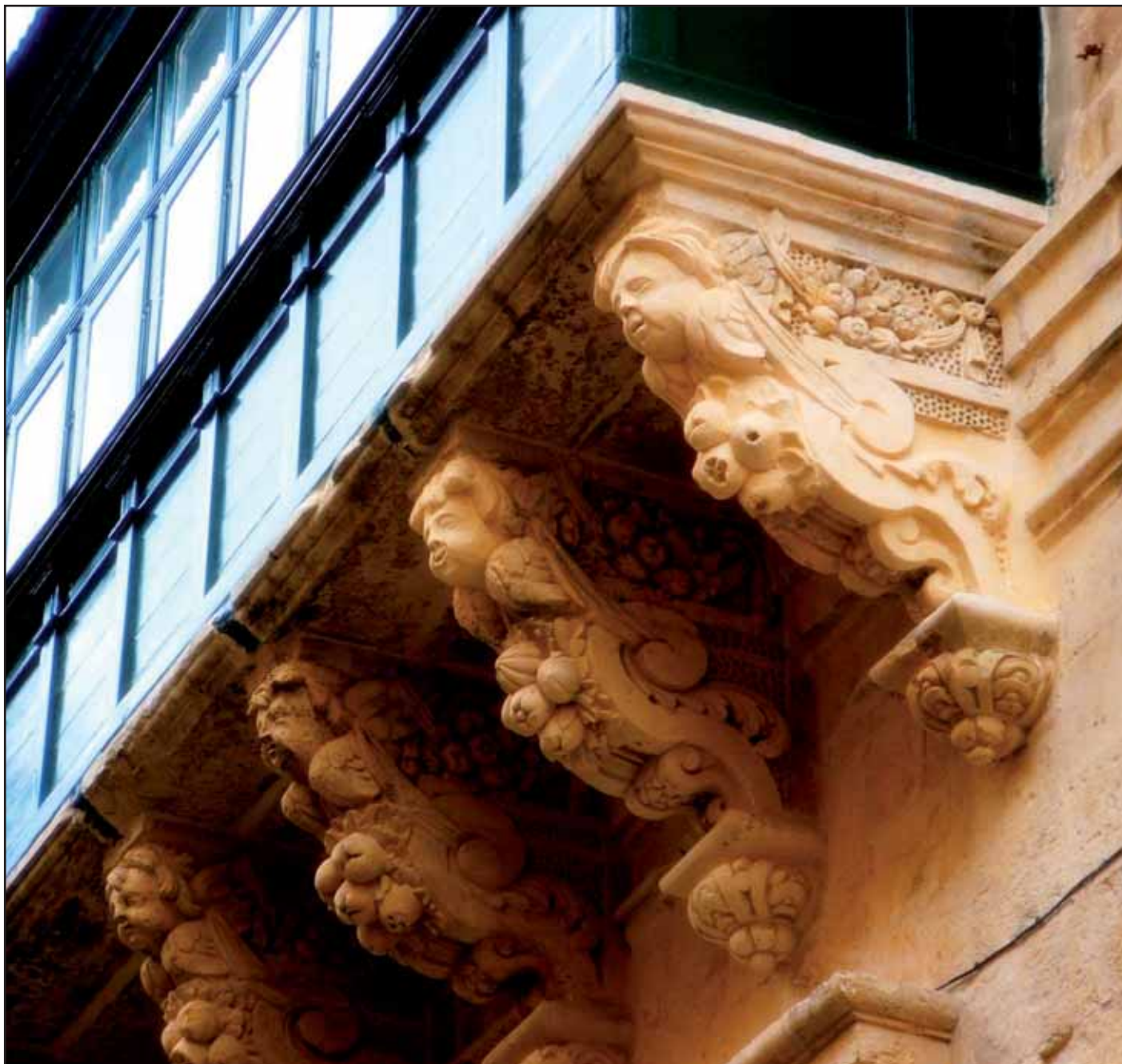
Recently restored balcony forming part of St John's complex
