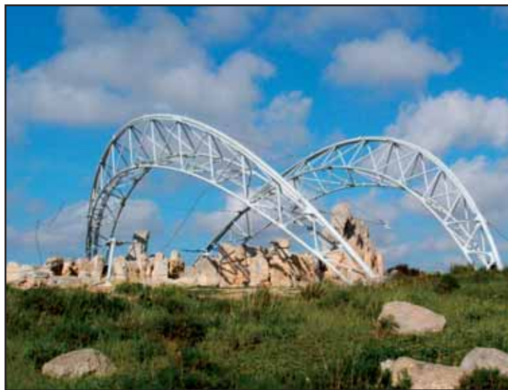
Supporting structures for Haġar Qim cover
