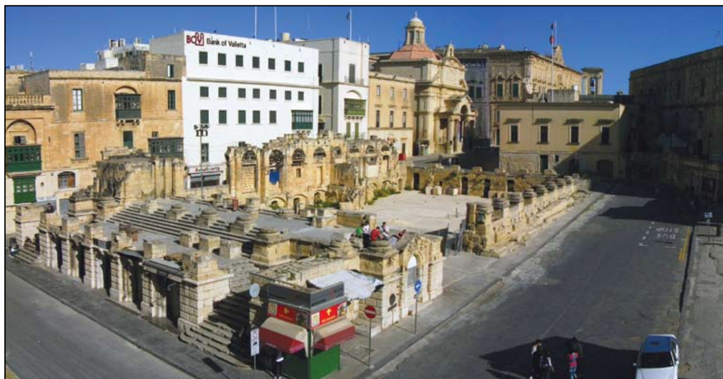
The project site before initiation of the project - Photo: David Cassar
