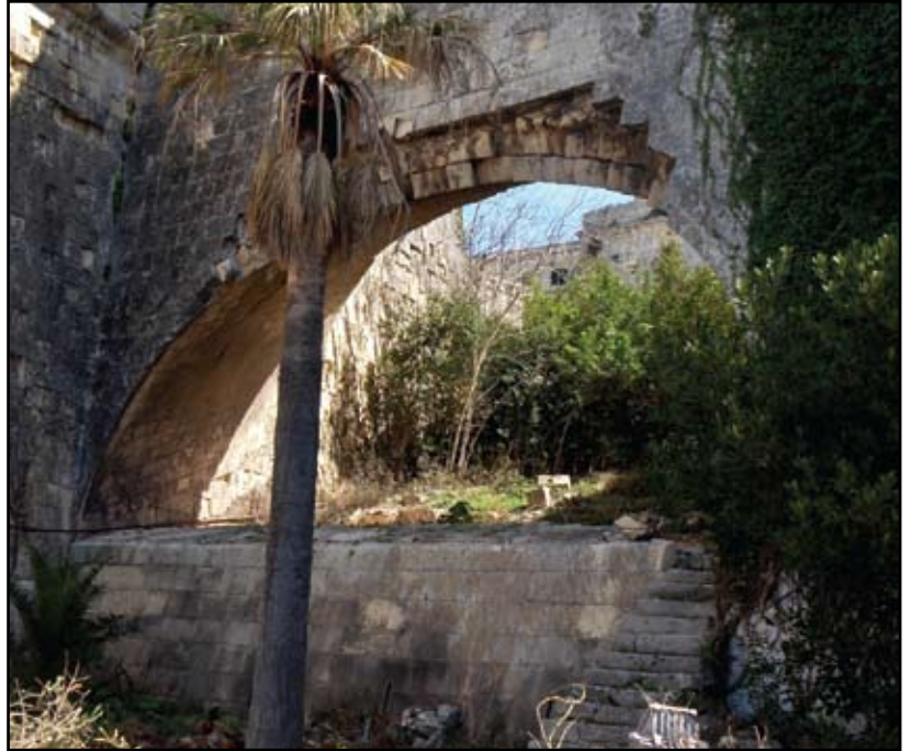
Literally falling to pieces. The unique skewed arch at il-Ġnien tal-Milorda (Sa Maison Garden). Photo - Victor Rizzo
