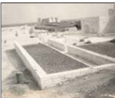
Building at San Tumas Point
