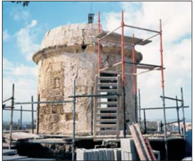
The Gardiola (Vedette) on St James' Bastion during restoration
