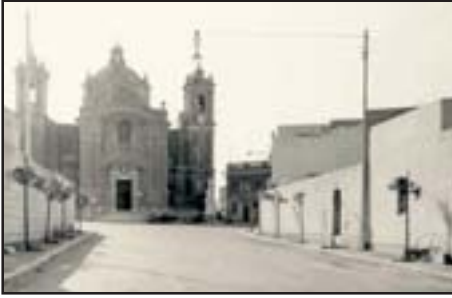
Newly cleared road in front of Qrendi parish church
