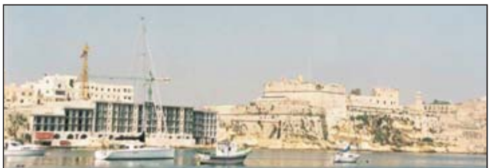
Building the Hilton tower and the new flats in Birgu
