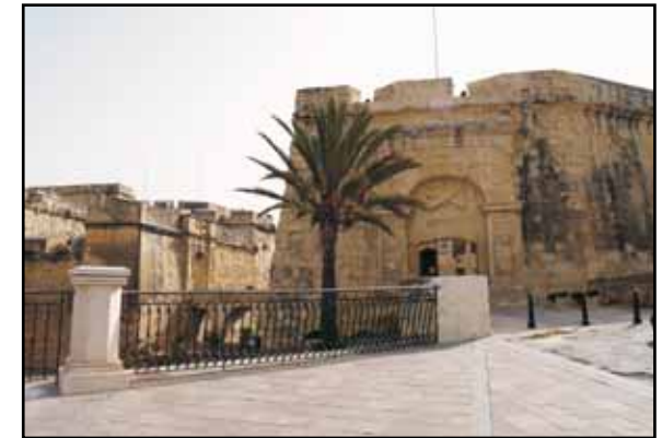
Advance Gate with Couvre Port in the background
