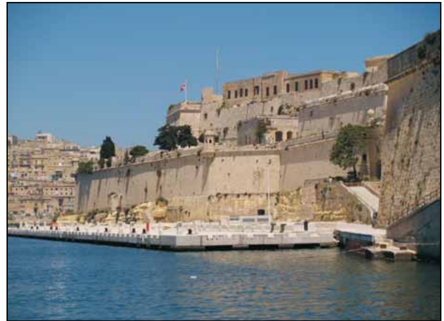
Fort St. Angelo - The Grunenburgh Battery
