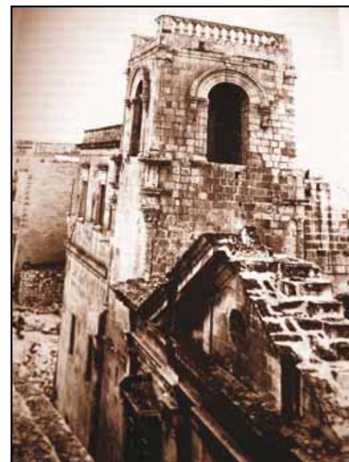
The lost Old Campanile
