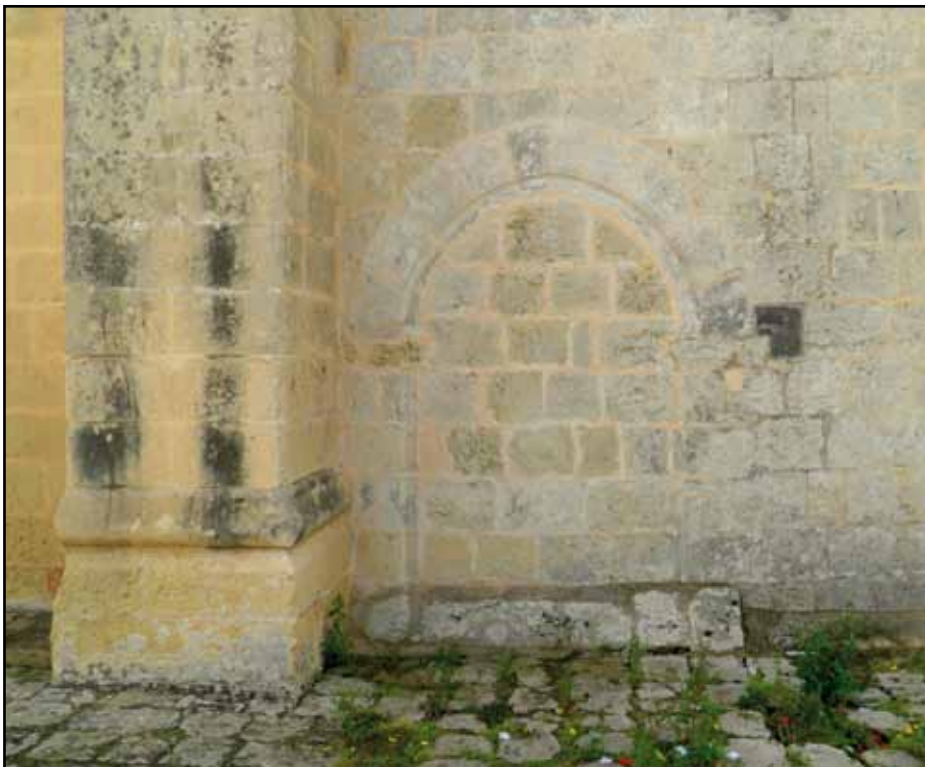
Blocked doorway formerly leading to the Bonici family chapel
