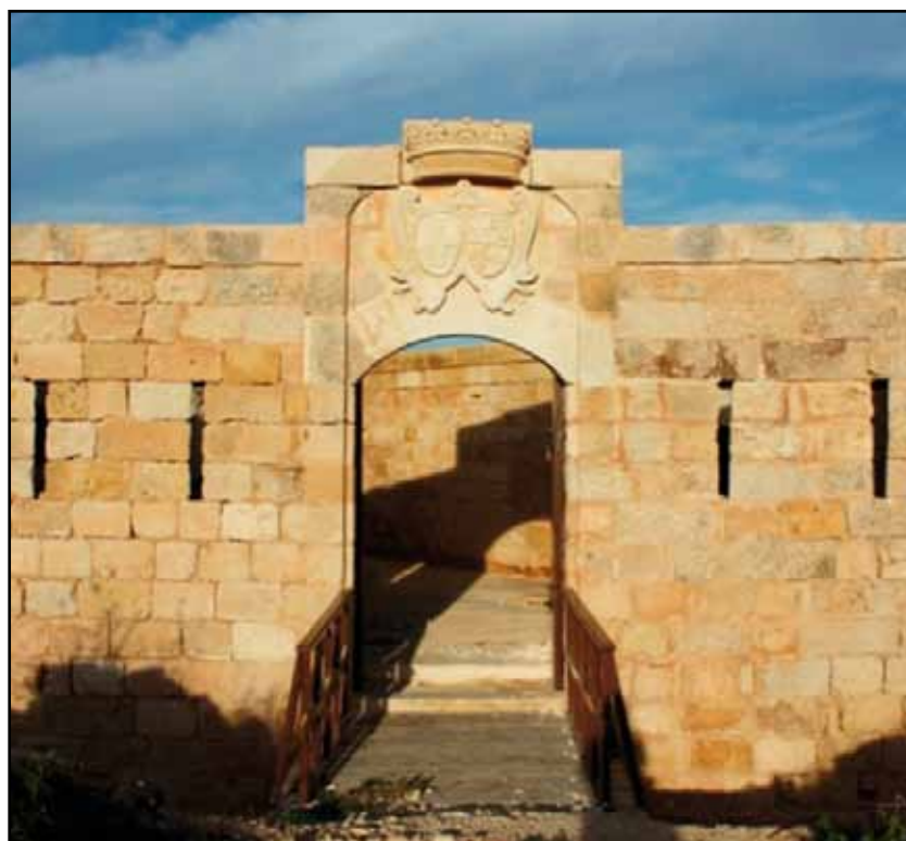
The restored entrance to St Anthony's Battery
