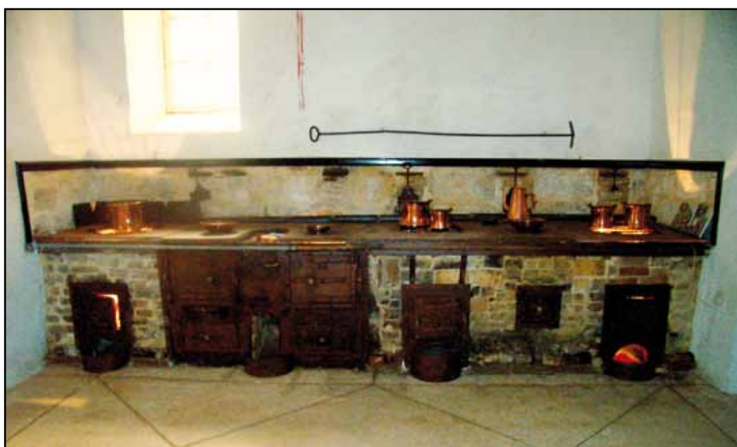
The Santo Spirito stove after restoration
