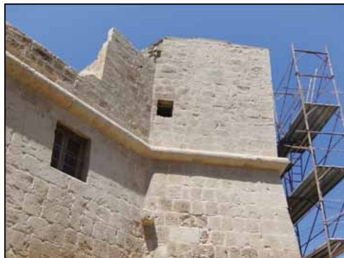
Mamo Tower undergoing restoration
