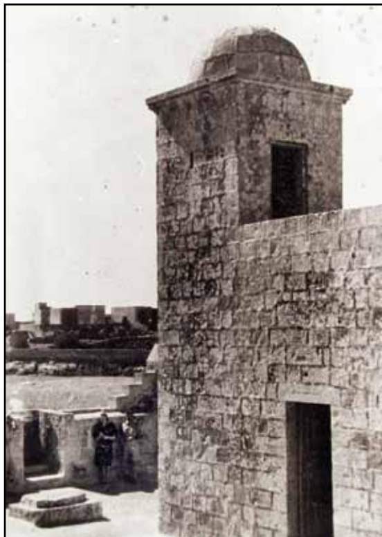
Detail showing the domed stair-hood. Photo courtesy of The National Archives, Gozo Section
