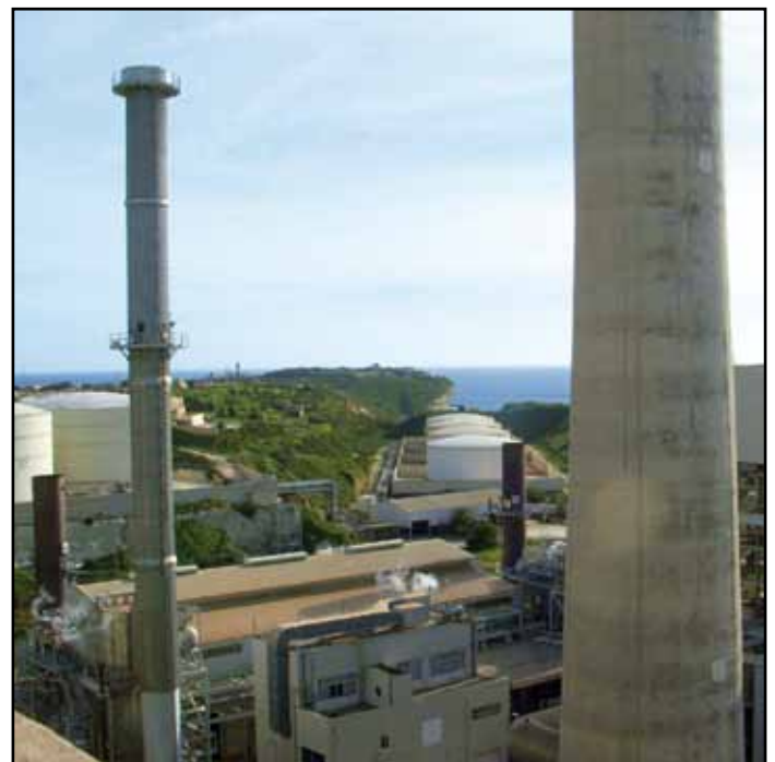
Details of the current Delimara Power Station
