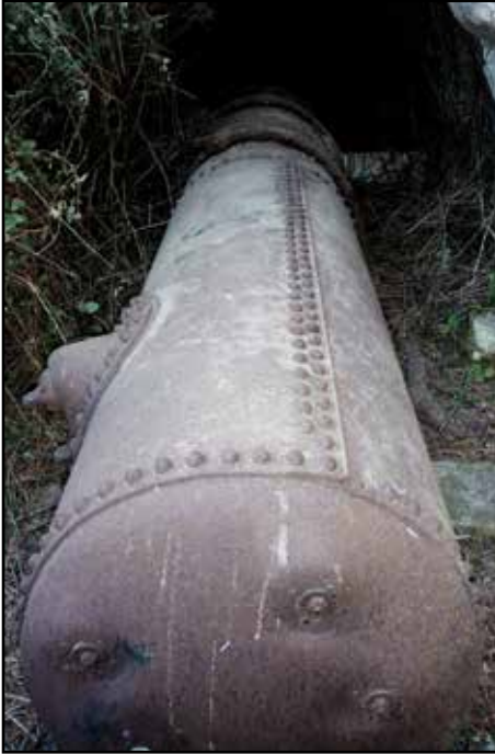
Part of the original pipe work on the bed of the valley
