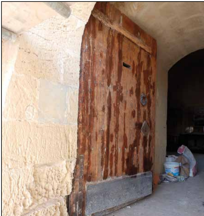
The red deal door after cleaning
