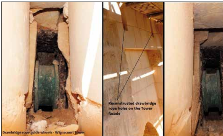
photo 1 - the drawbridge guide wheels
