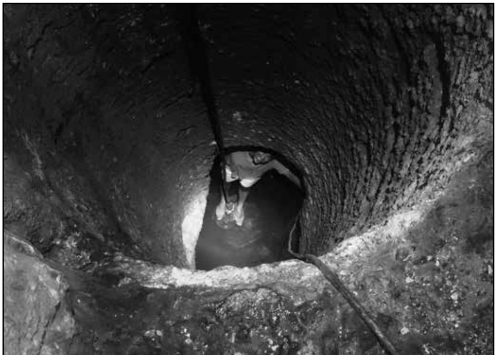
The underground pit hosting the pump
