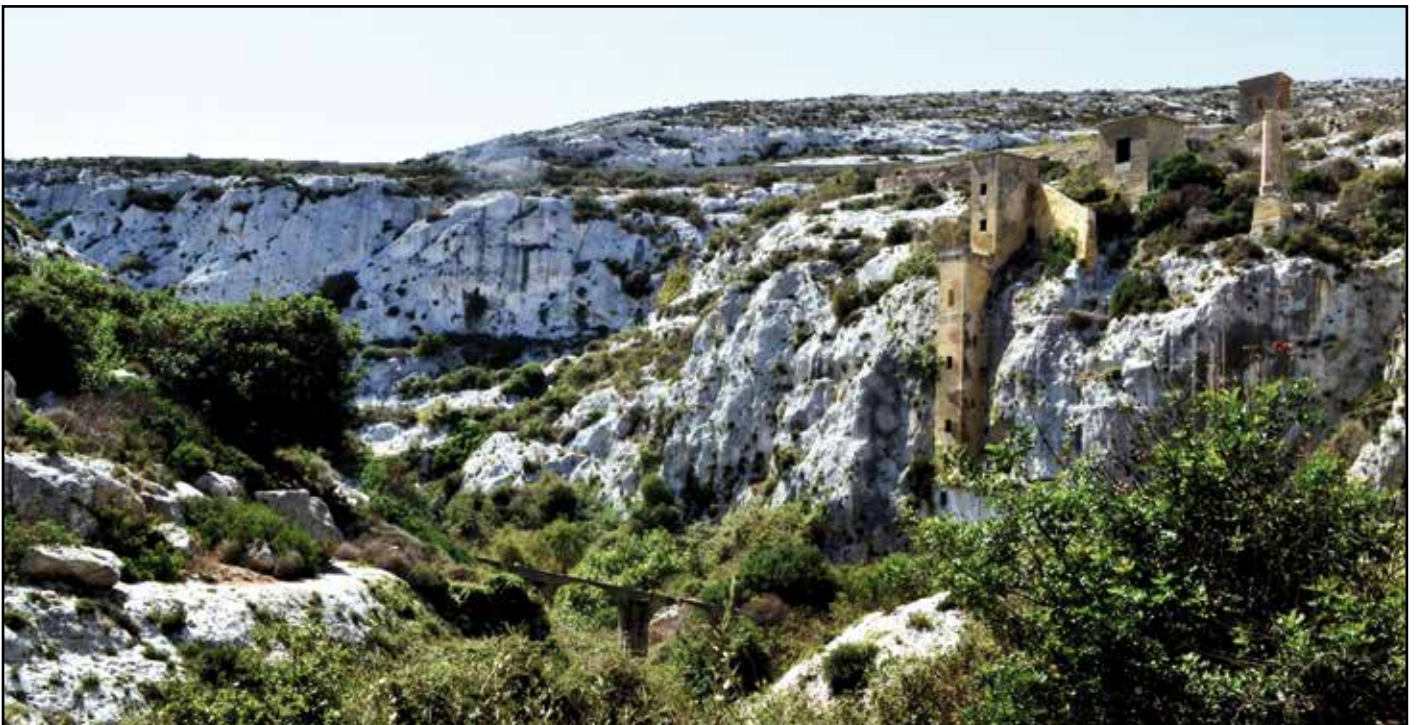
The pumping station in its current state
