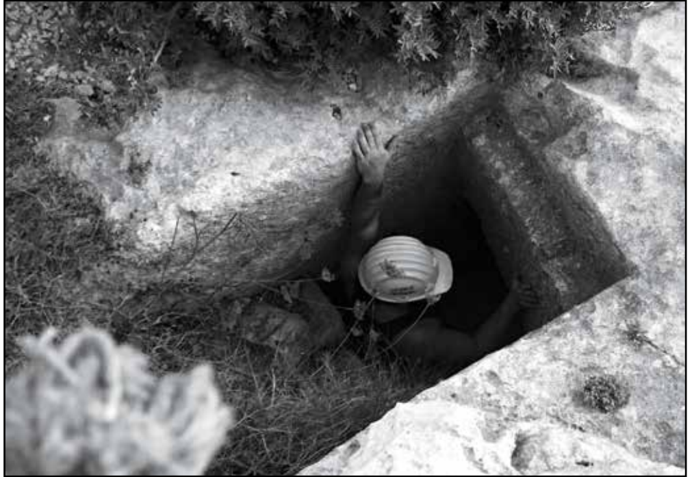
The tunnel which used to host the pipeline to the Nadur Reservoir
