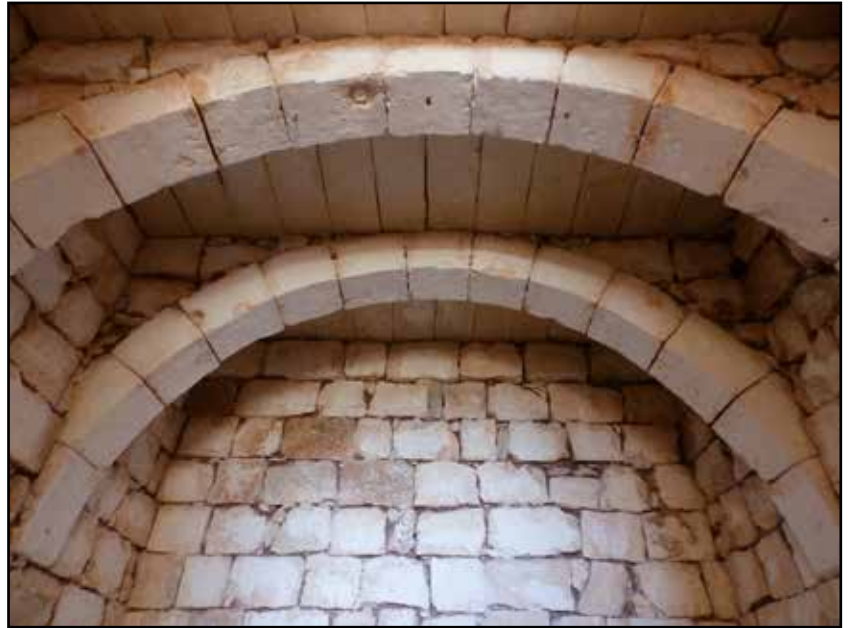
The interior of the lower floor of the tower after cleaning
