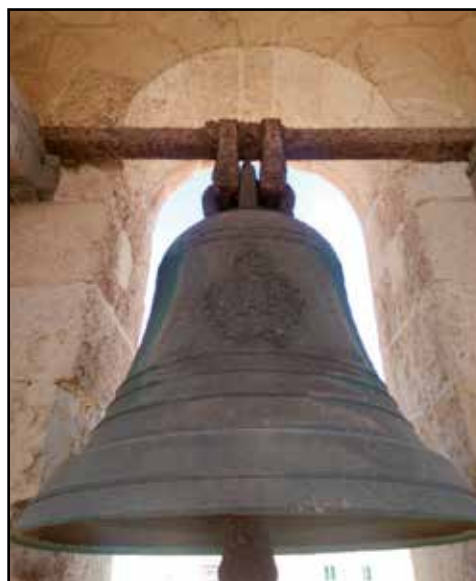
Showing corrosion to the cross bar and damage to stone work
