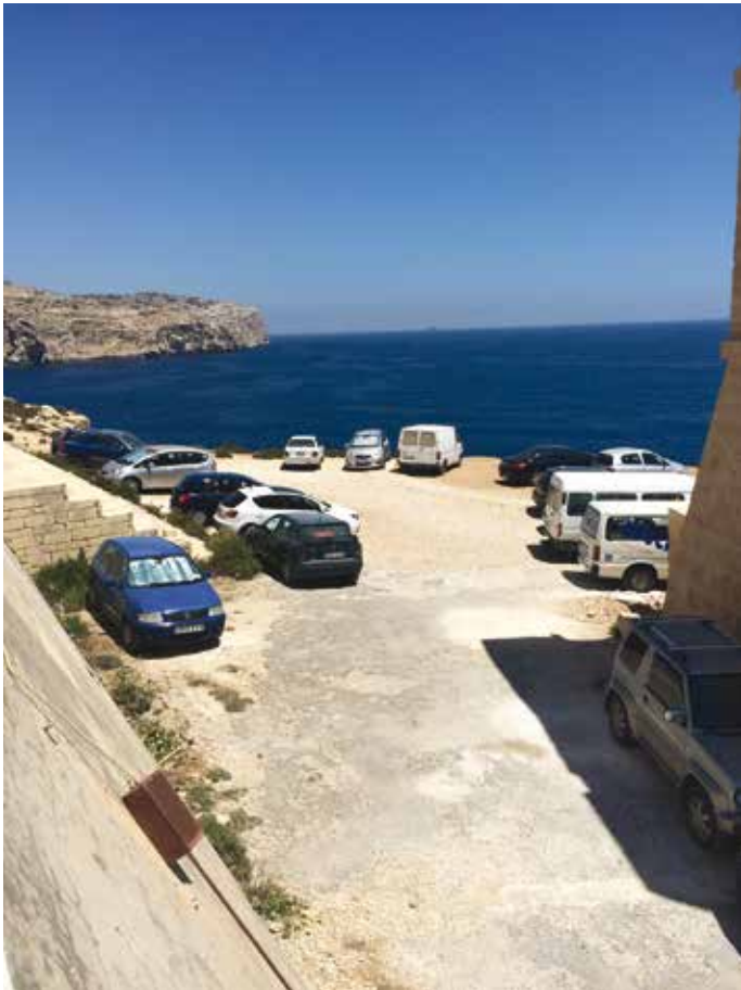
The dismal state of the surroundings before restoration
