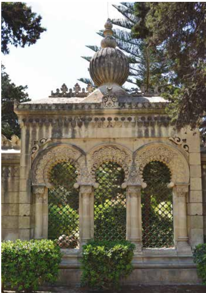
The main jali screen window that forms part of the front façade (Photo: Conrad Thake)
