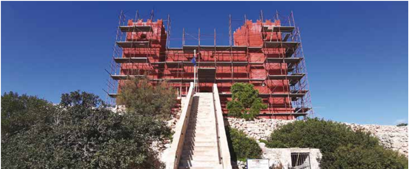
Red Tower façade under restoration
