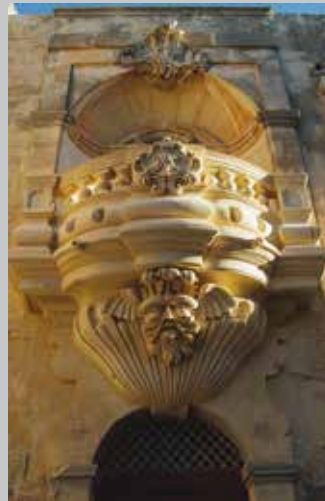
No 34 Main Street, Lija, winner of a DLH Diploma for Restoration and Conservation
