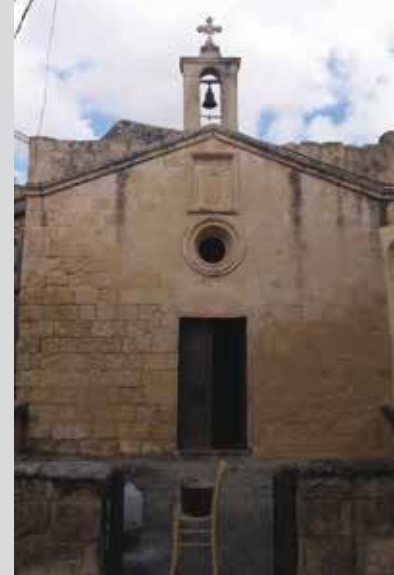
St Roque Chapel facades being restored
